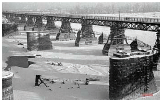
Fig. 5. Temporary bridge with visible supports of demolished railway bridges by the Citadel. Supports of the older bridge have been rebuilt just after the war, but the bridge itself was rebuilt only in 1959...
